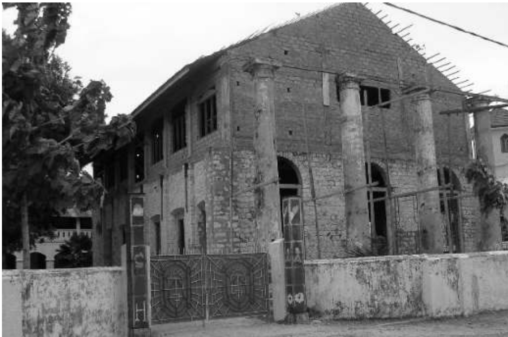
Romaine Hall under Renovation
